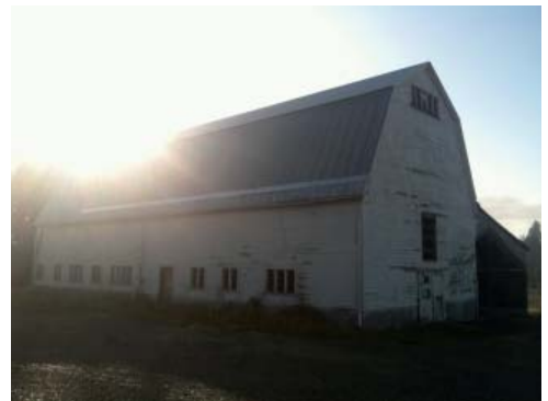
North side of barn
