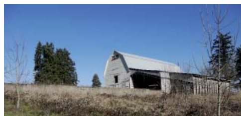
Barn and Accessory Shed Additions
