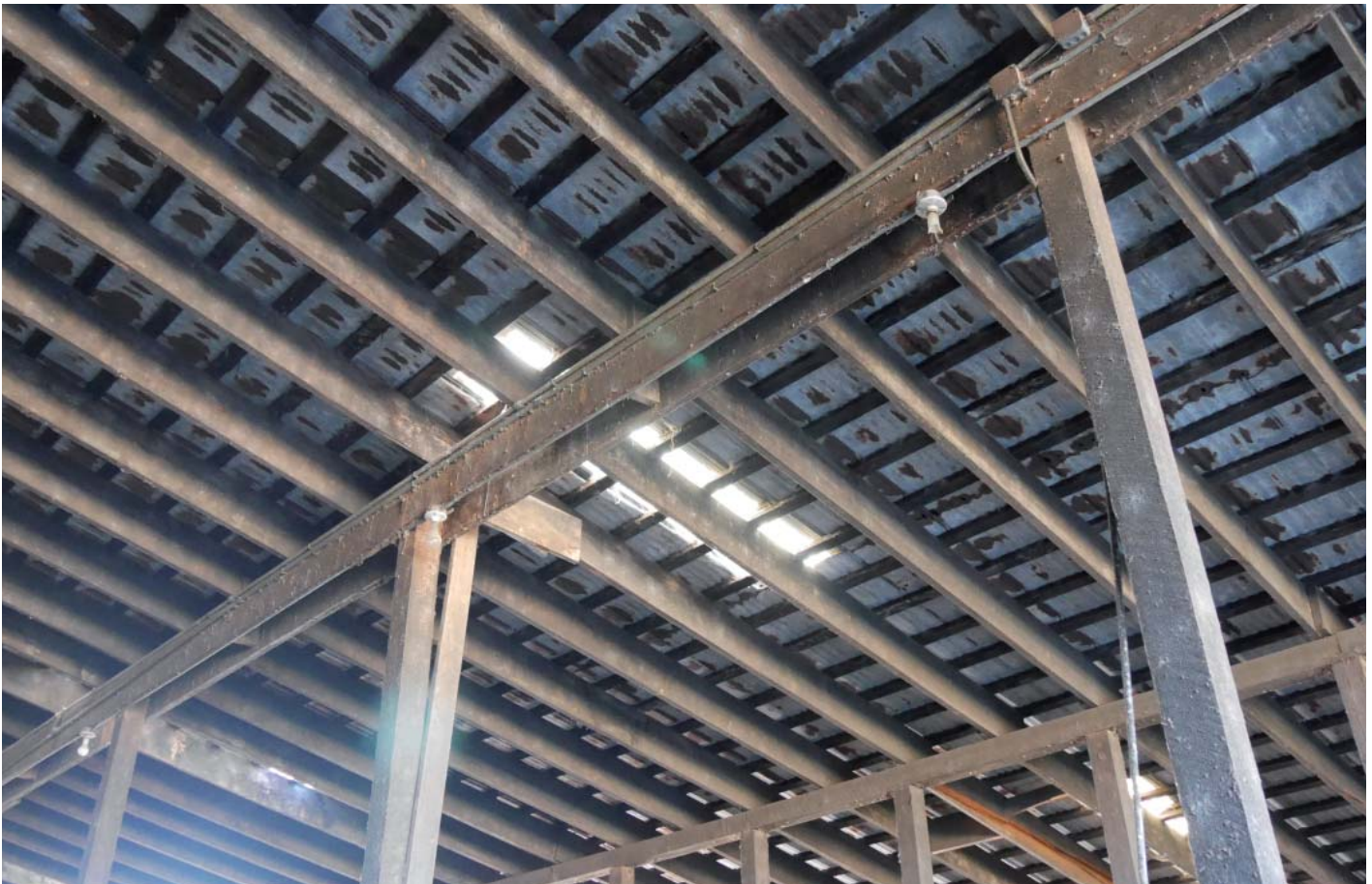
Wood and roofing for salvage
